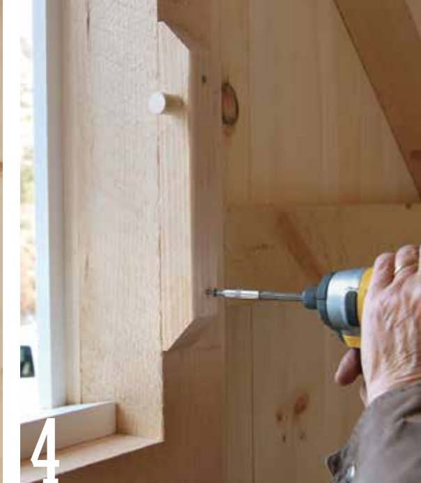
4 Mount a stop to each side of the windows. When the sash is open, it'll rest against the wood dowel protruding from the 2×2 cleats.
