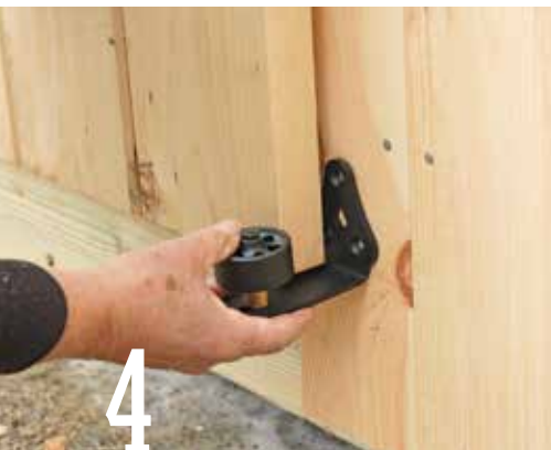
4 To keep the sliding door from swinging away from the barn, attach a stay roller to the barn near the bottom corner of the door.
