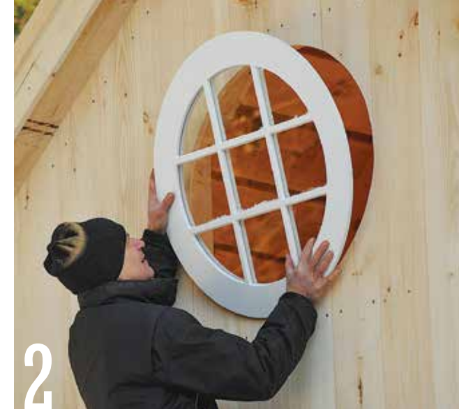
2 Tilt the round window into the opening, then level it. Secure the window by driving four 2½-in. screws through its perimeter flange.
