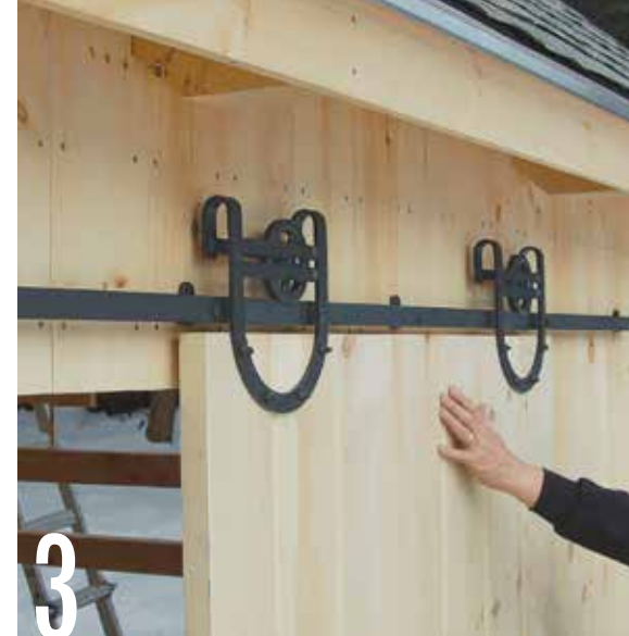
3 Slide the barn door onto the tracks. Each roller assembly houses a grooved wheel. Be sure the grooves fit over the top of the track.
