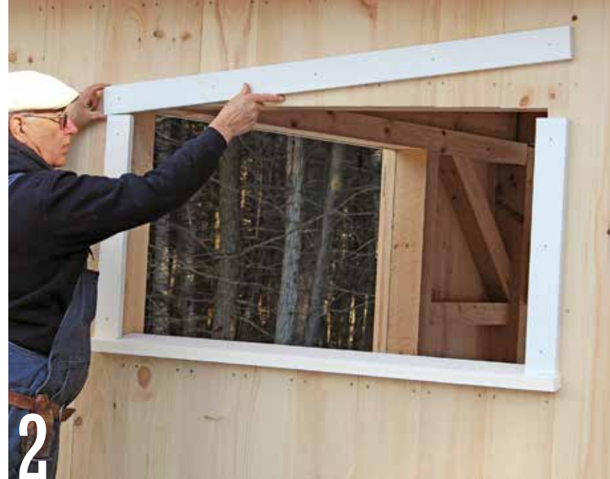
2 After attaching both side casings, install the head casing across the window top where it, too, will protrude ¾ in. into the opening.
