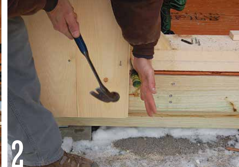
2 If a siding piece is bowed and you can't tighten the joint, pry it closed using a wood chisel hammered into the timber frame.
