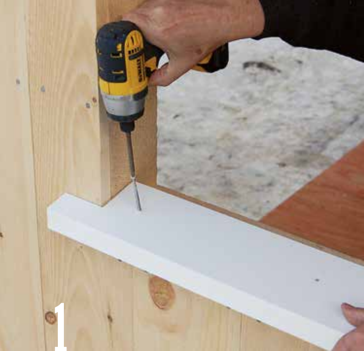
1 Fasten the sill into the window opening with 2½-in. trim-head screws. The horn on each end of the sill extends 3 in. past the opening.
