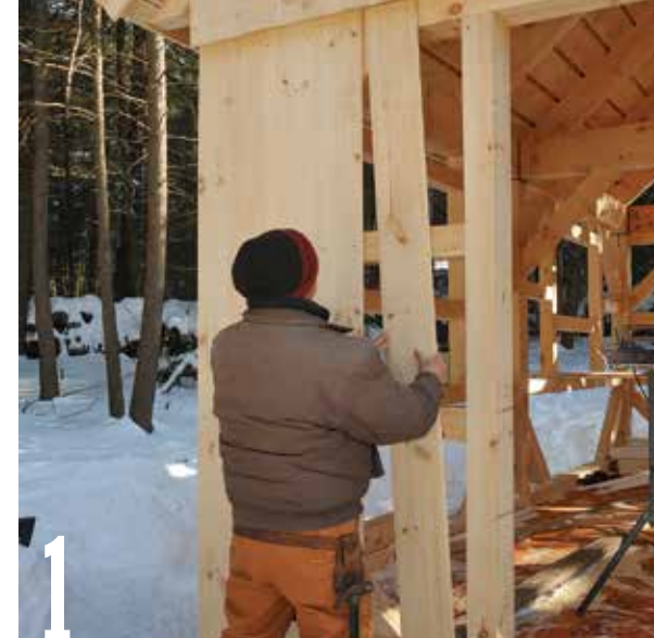
1 Install 1×8 pine siding across the gable-end wall. Slip each piece under the siding above and secure with 2½-in.-long galvanized nails.
