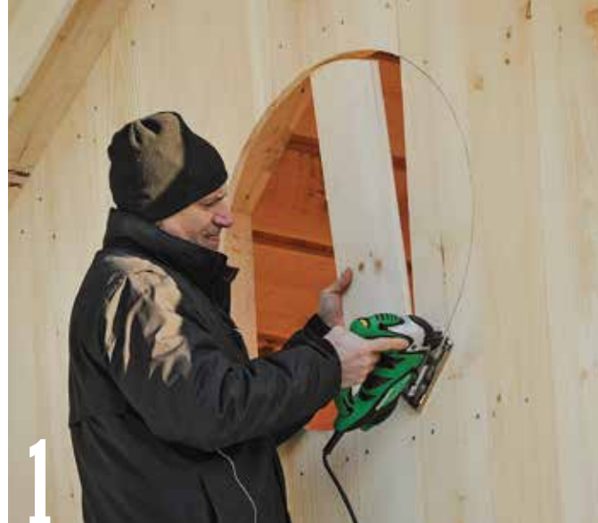
1 After marking the round window opening onto the gable end, use a jigsaw to cut the 30-in.-dia. circle through the 1×8 pine siding.
