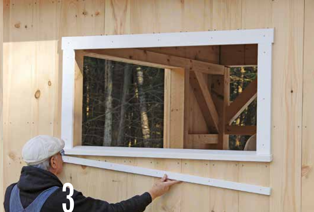
3 Install the apron under the windowsill, attaching it with 2½-in. screws. Conceal all screw heads with white caulk or plastic plugs.
